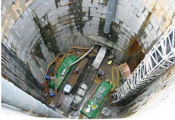
Figure 6-7: Intermediate Shaft for PTP System [128].
