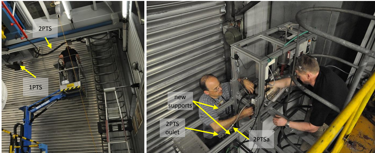
Figure 43 Installation of section 2PTSa into test cell
