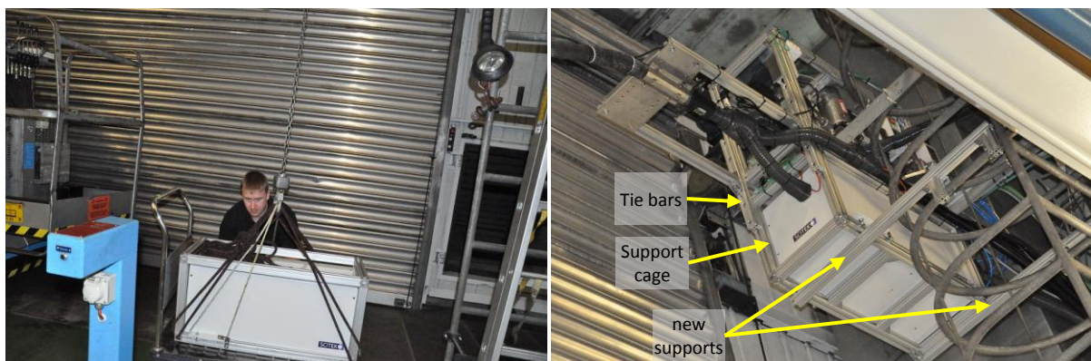
Figure 44 Installation of 3PTS section into SR Technics test cell
