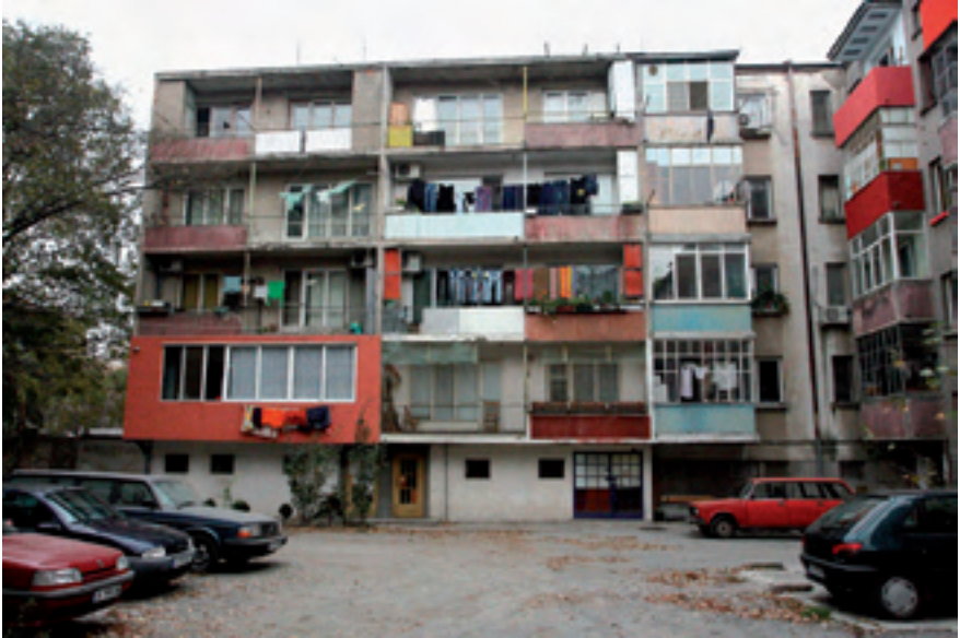
Picture 8. One of the many buildings in the UNECE region waiting for retrofitting measures
