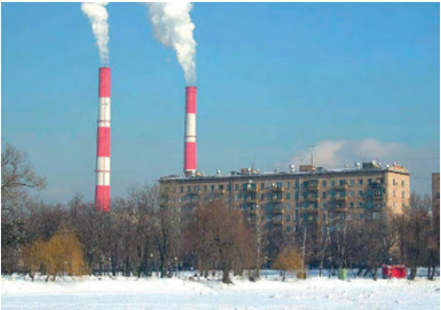
Picture 6. A power station overlooking housing estates in Moscow, February 2009
