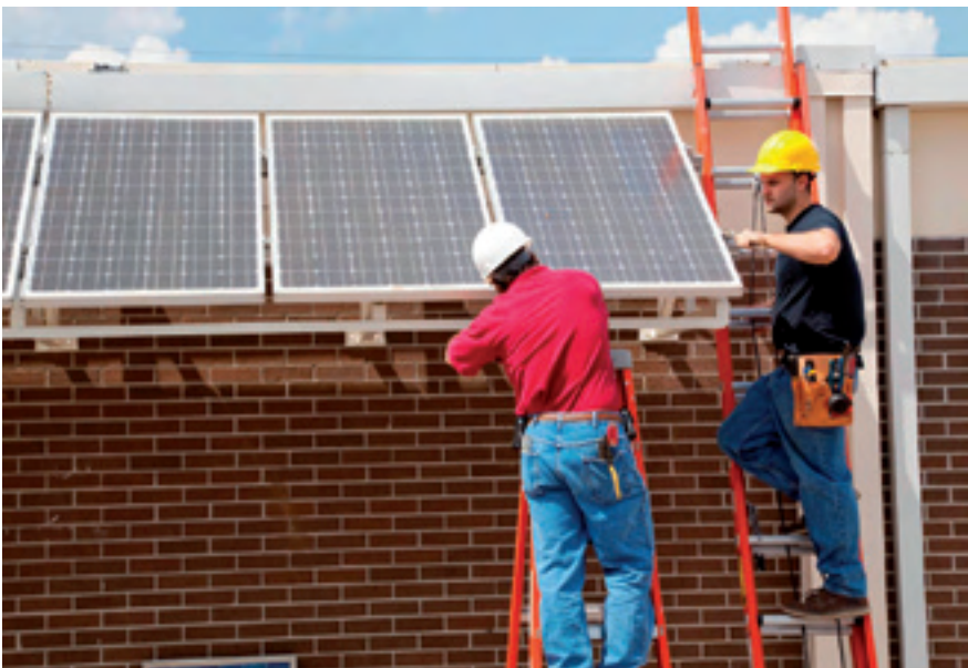
Picture 4. Workers installing solar panels in Eastern Europe.
