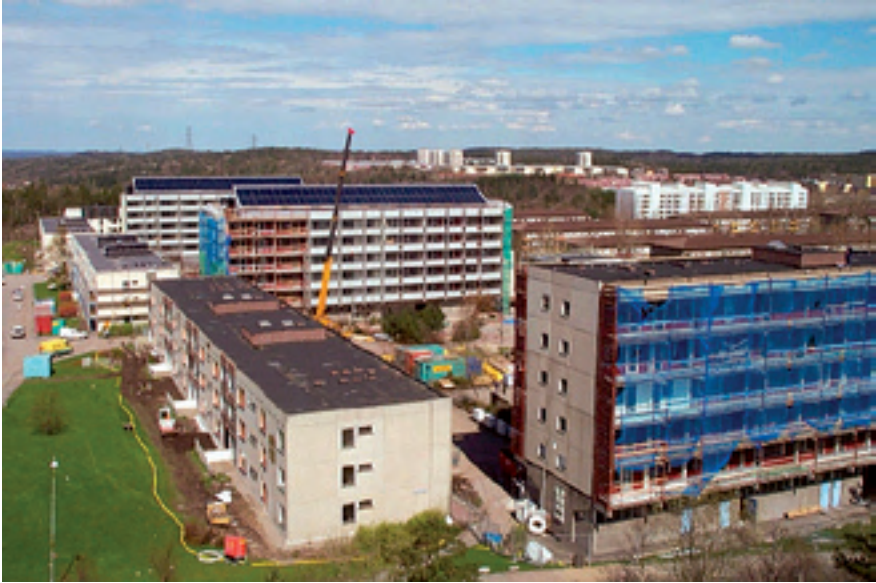
Picture 3. In Gardsten, Sweden, 1400 m 2 solar panels provide energy for some 500 flats.
