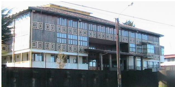
Figure 22. School G, External view
