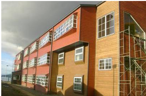
Figure 24. School H, External view
