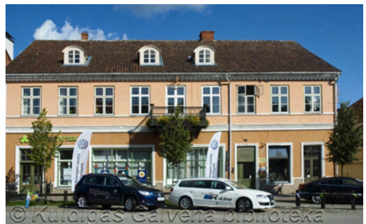
Figure 3 – Kuldīga town centre – a library building
