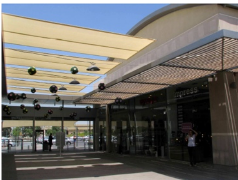
Figure 2: All circulation areas are shaded by a combination of pergolas and removable fabric awnings.
