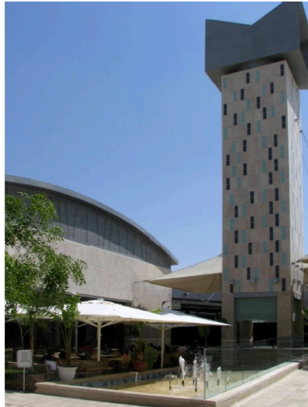
Figure 5: Cafes in the two plazas enjoy evaporative cooling from small fountains and from a downdraft cool tower.
