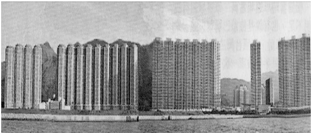
Figure 1: An example of wall building on the waterfront in Hong Kong
