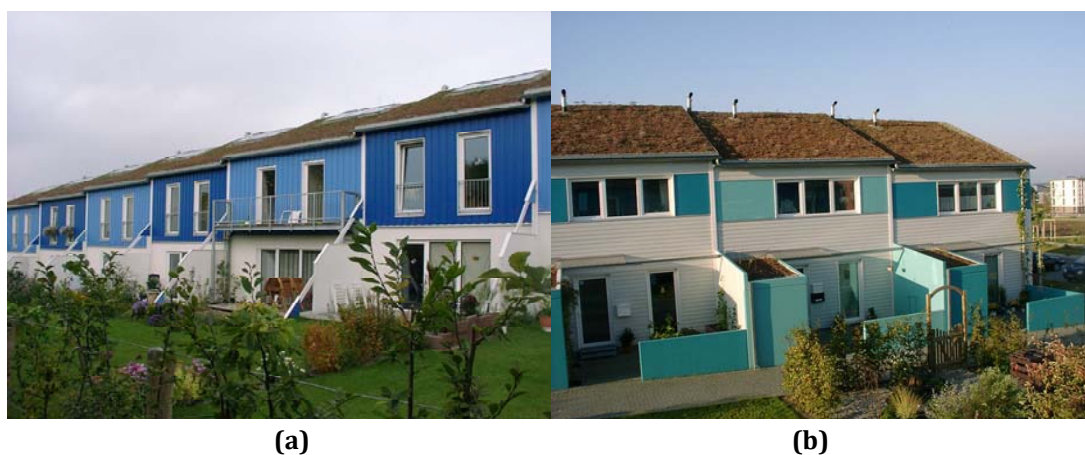
Figure 6.1 The (a) south and (b) north façades of the terraced buildings in Hannover Kronsberg (Feist et al. 2001)
