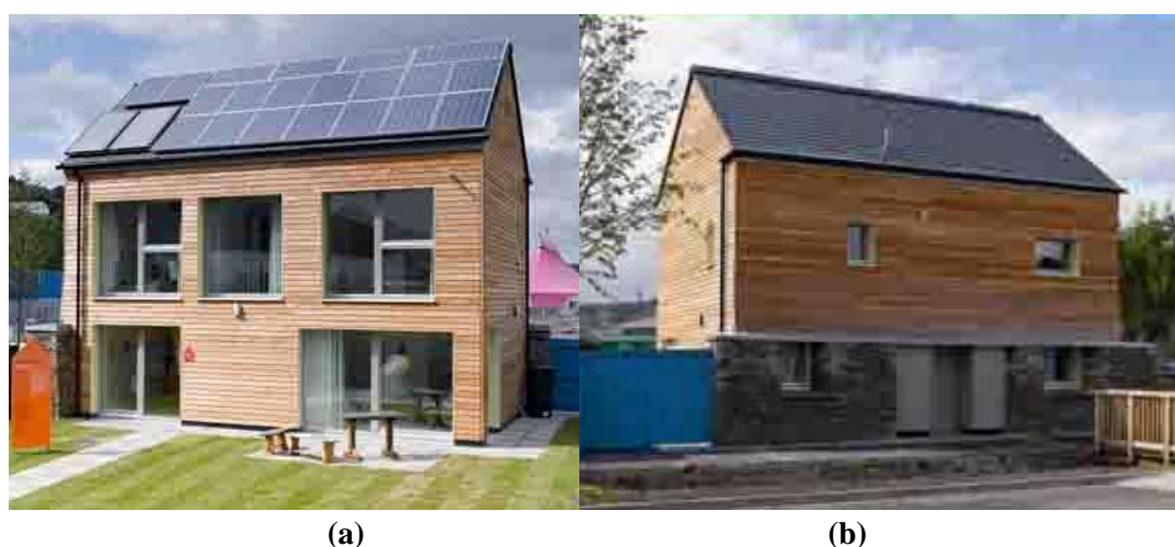
Figure 6.10 Views of the Larch House, from the (a) South and (b) North (iPHA 2012b)
