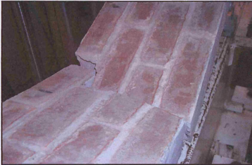
Plate 5.7- Failure in prototype flexural strength specimens.
