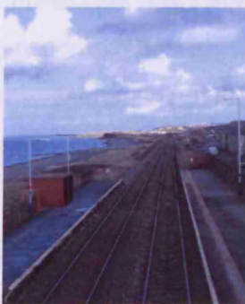
Workington, Network Rail
