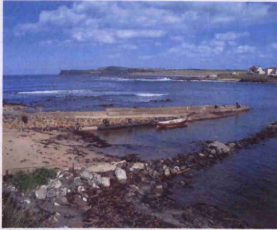
Leslie's Pier (north western section of bay)
