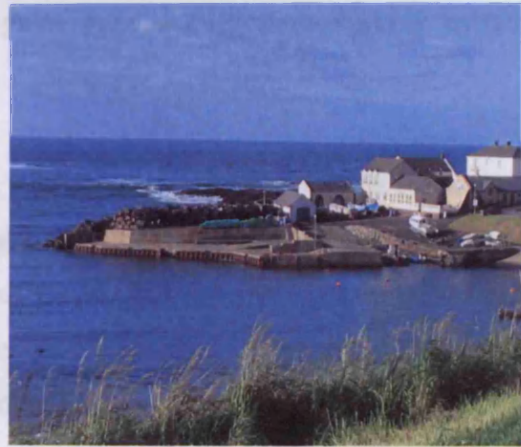
Portballintrae Harbour (eastern section of bay)
