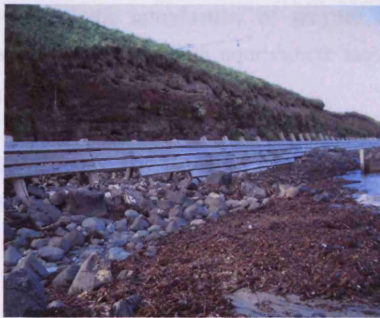
Retaining wall (western section of bay)
