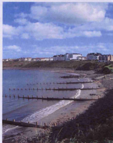
Groynes (south western section of bay)
