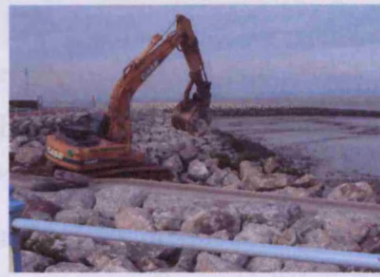
Morecambe, Lancaster City Council
