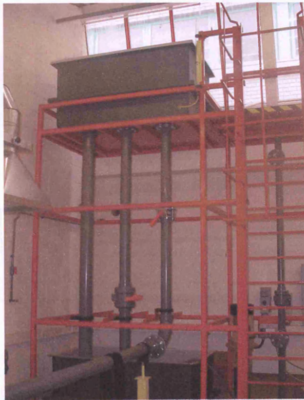
Figure B2. The stand, header tank and inlet pipe to the 0.75m diameter Grit King ® in the laboratory at Cardiff University.
