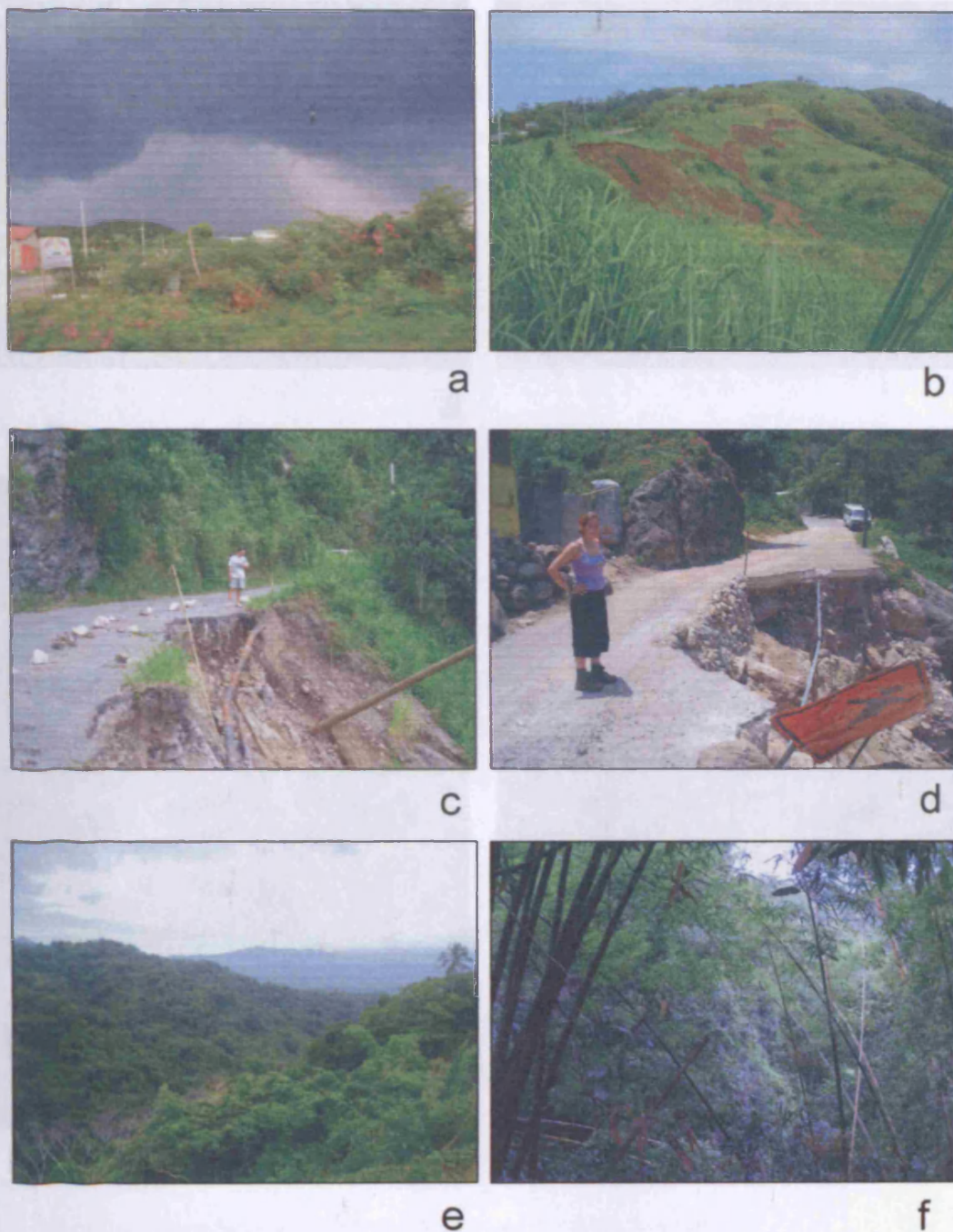
Figure 4.1 – (a) Tropical storm over the Central Inlier; (b-c) Landslide in the Central Inlier caused by a tropical storm, such landslides cover outcrops (c-d) Roads were washed away by torrential rain brought by hurricane Emily on the 17 th July, 2005. These two examples were found whilst attempting to reach outcrops of the Bath-Dunrobin Formation in 2005; (e) Most of the interior of the island is made up of dense forests and hills; (f) On foot it is apparent how thick the vegetation can be in many places.
