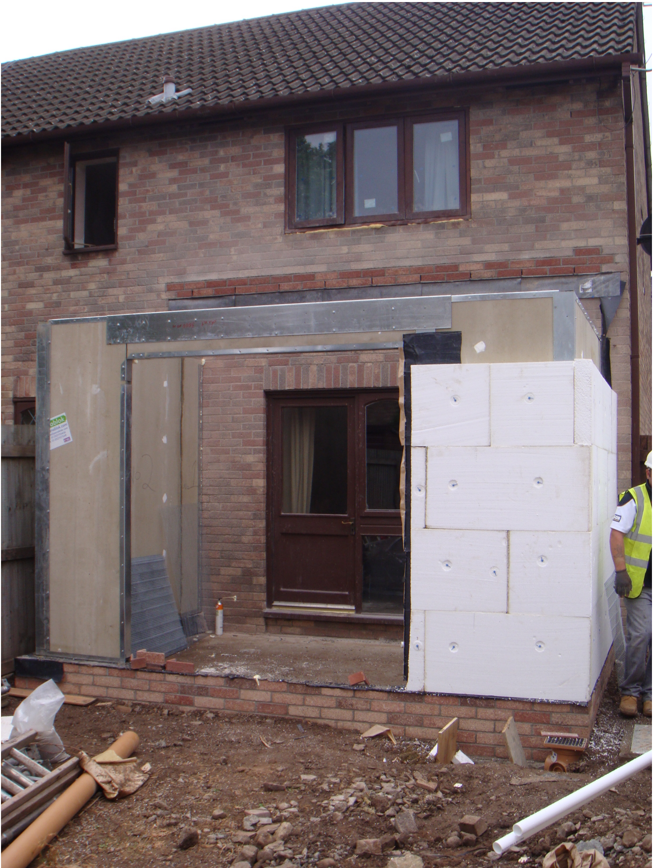
New conservatory space constructed using prefabricated walling elements
