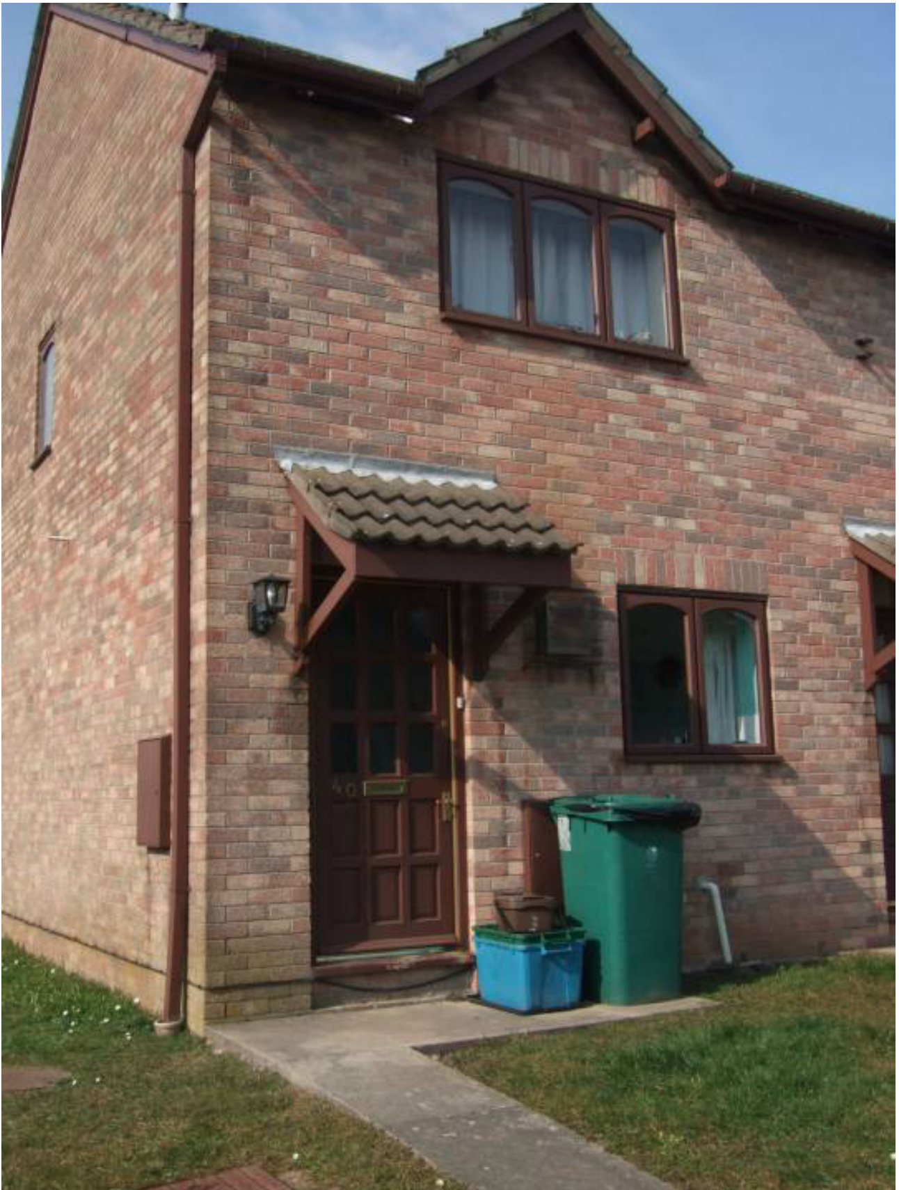
The existing end of terrace house
