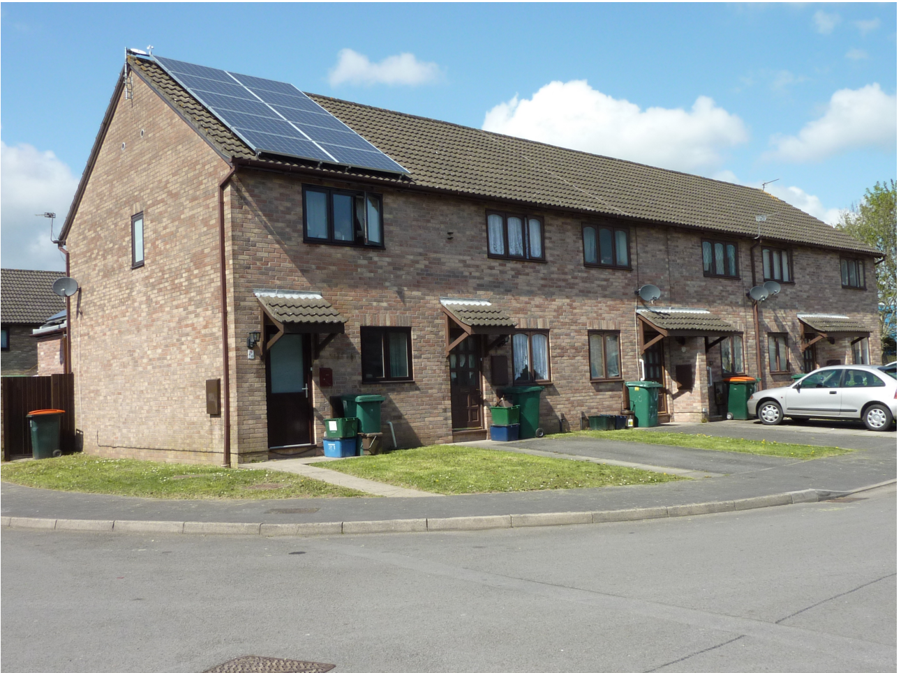
End of terrace retrofit
