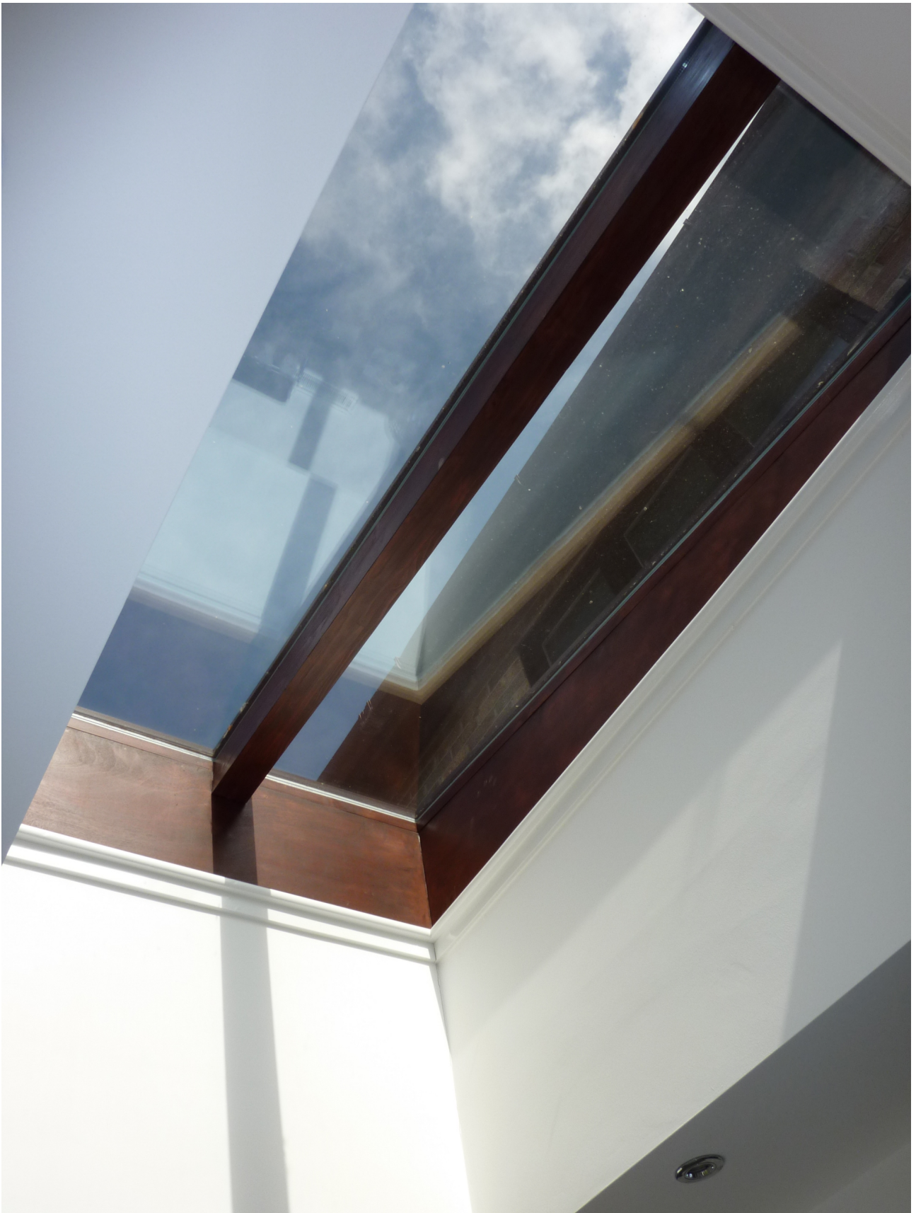
Rooflight to maximise day-lighting over conservatory
