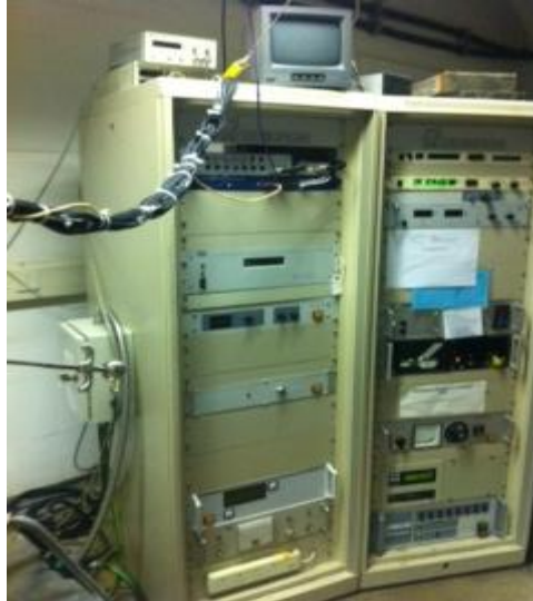
Figure 4.2: Control towers of the UHV system
