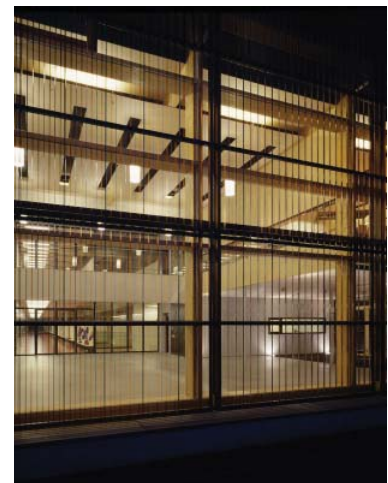
Copper 'veil' as seen from the South during the day (top) and evening view with lit interior visible through the perforations.
