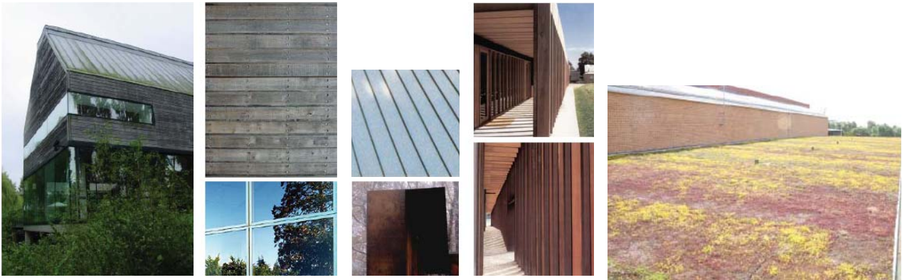
Figure 22 Original palette of materials – weathered hardwood cladding, open walkways, sedum and metal roofs - designed to blend into landscape
