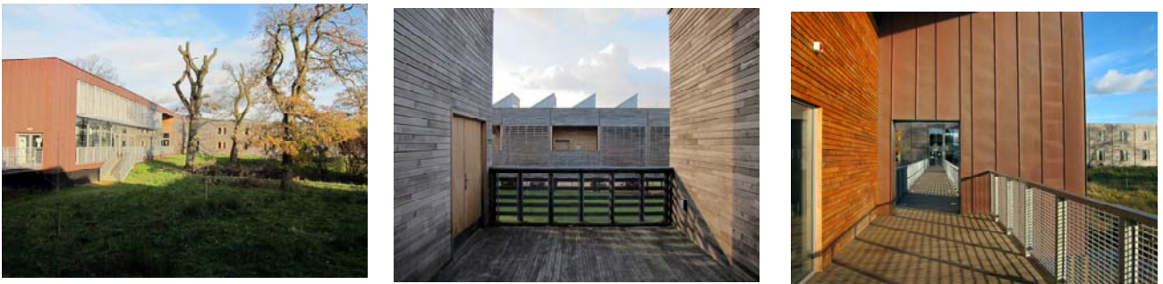
Finished building showing predominant materials – Sweet Chestnut Cladding, Pre-patinated copper
