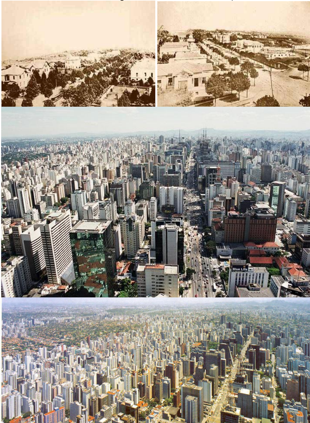
Figure 5-22: Paulista Avenue, at the turn of the 20 th century (above); and nowadays: a high-rise tower urban corridor in the city of São Paulo (general view at top-middle and middle-bottom, and schematic longitudinal section at the bottom).
