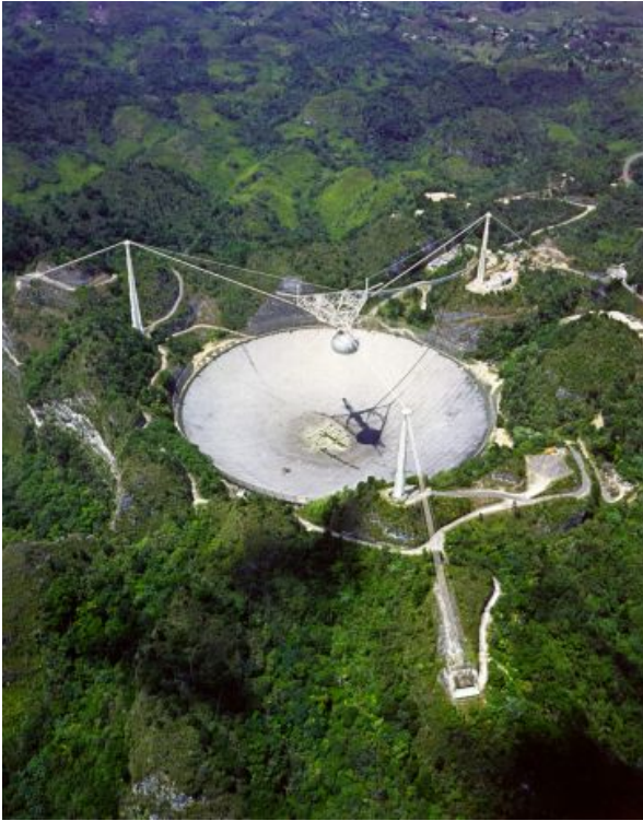
Figure 1.1: Arecibo Radio Telescope — The 1000 ft. (305 m) diameter telescope, located in Puerto Rico, is the largest single-aperture telescope ever constructed. It collects radio waves that are analyzed by the SETI@Home software. Some might recognize it as the setting for the end-scenes in the James Bond movie “Goldeneye,” as well as a good portion of the movie “Contact.”
