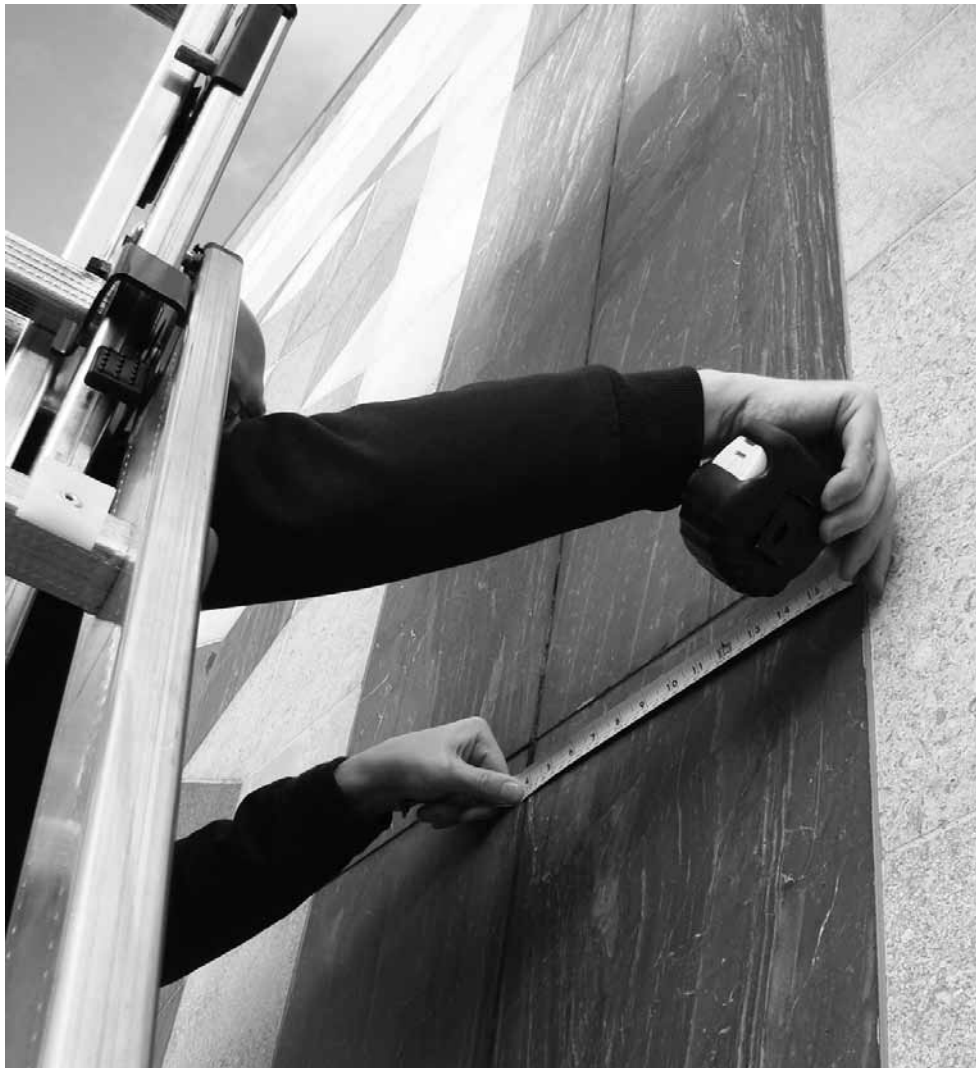
9 Measuring the constructed joints on the west elevation, Caruso St John Architects' Victoria and Albert Museum of Childhood entrance addition
