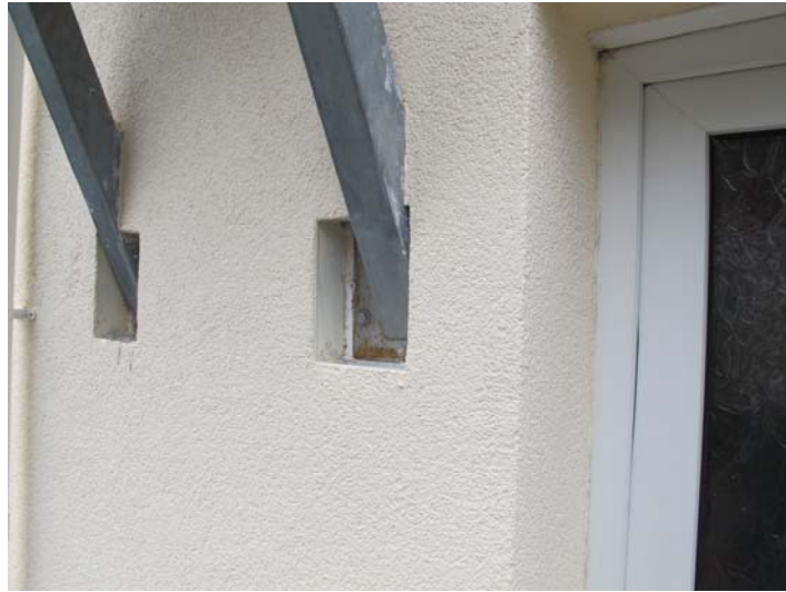
Figure 4.11 - Detailing around balcony support brackets
