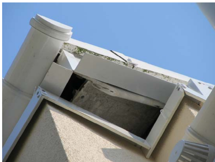
Figure 4.8 – Complex detailing around the roof line
