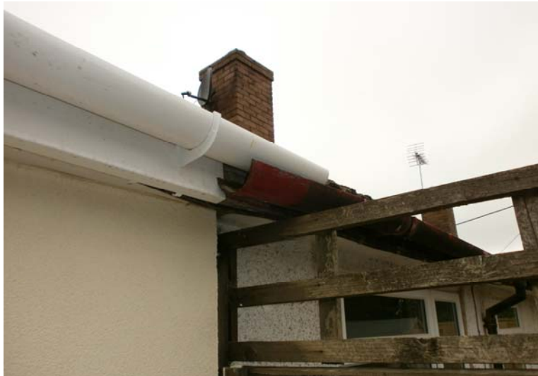
Figure 4.21 – Undertaking works on adjacent properties
