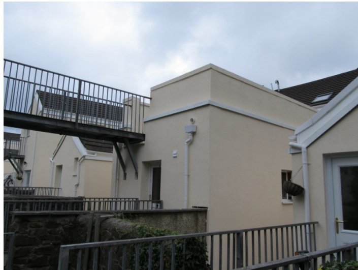
Figure 5.10- Complexities of detailing when installing EWI
