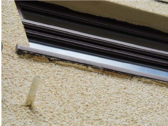
Figure 4.17 - Rendering under the sill
