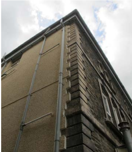
Figure 4.7 – Dealing with detailing when installing EWI
