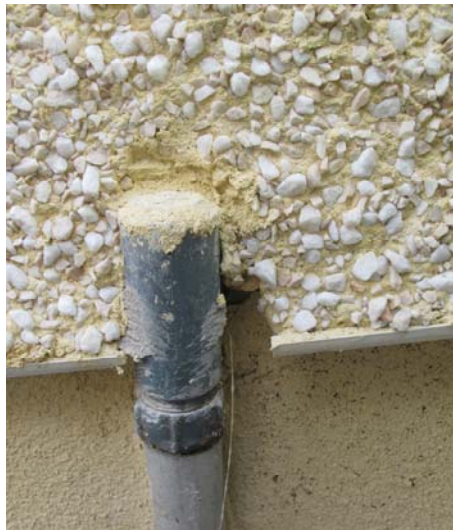
Figure 4.14 – Detailing around services entering a property
