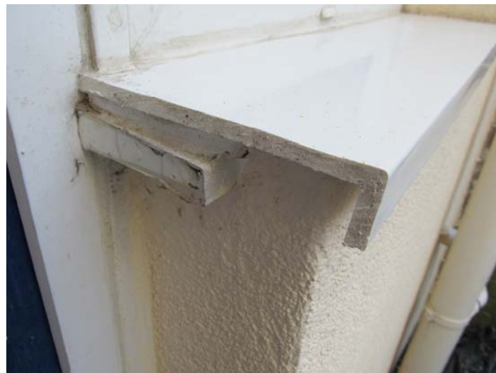
Figure 4.16 - Fitting a new sill over existing sill
