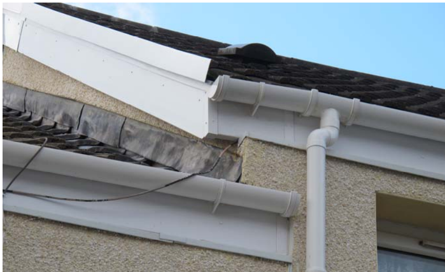
Figure 4.20 – Junctions between properties on a steep road
