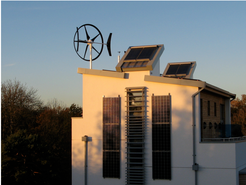
Figure 2: The Stewart Milne Group's Sigma Home at the BRE Innovation Park, Garston—low energy design introduces new appearances and ways of operating a home.
