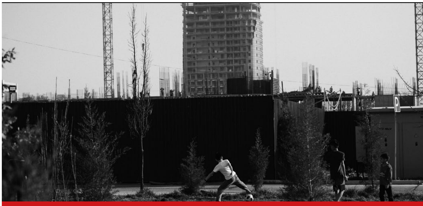
Image 4: Construction activity Tashkent City
