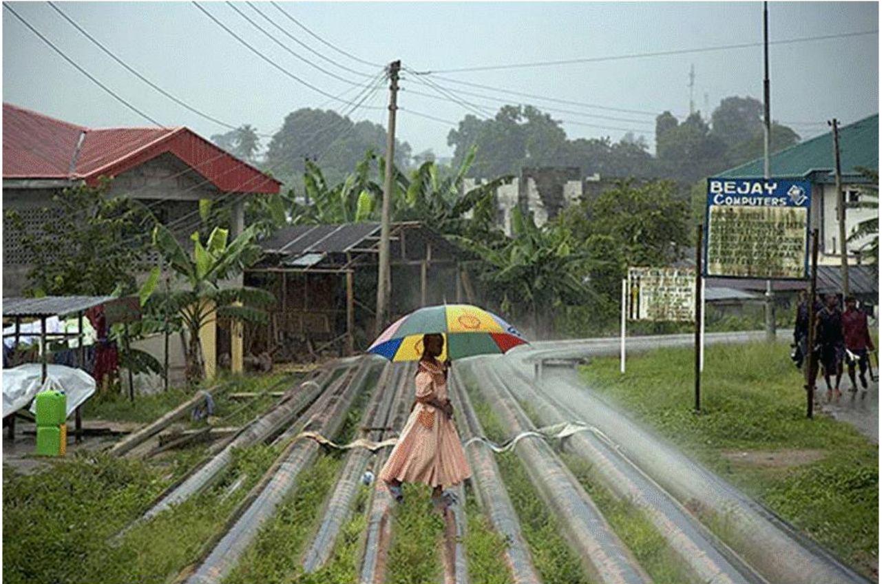
Figure 1. Pipeline ROW encroachment site (The Guardian 2005)
