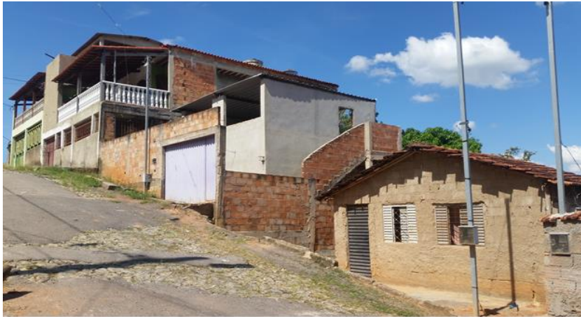
Figure 8. Nova Contagem neighbourhood: an almost original house in the bottom right of the picture and three rebuilt houses on the top of the hill
