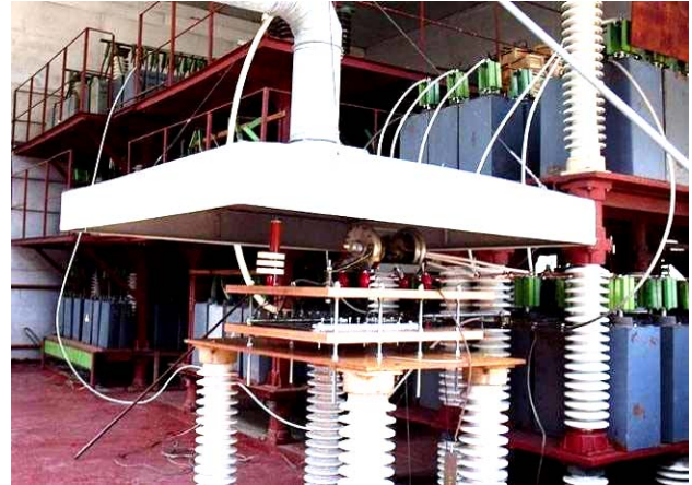
Fig. 2. General view of a high-voltage high-current test facility of the type UITOM-1 (developed by the Scientific-&-Research Planning-&-Design Institute «Molniya» of the National Technical University «Kharkiv Polytechnic Institute») which simulates the direct effect of the main components of the artificial lightning current on the TS of the metal panel of a domestic aircraft's fuel tank (in the foreground is a desktop with a three-electrode controlled air switch for voltage of \pm 50 \text{ kV} and an air exhaust system, and in the background are powerful high-voltage generators PCG-A, PCG-D, PCG-B, PCG-C and PCG-C*) [5, 6]
