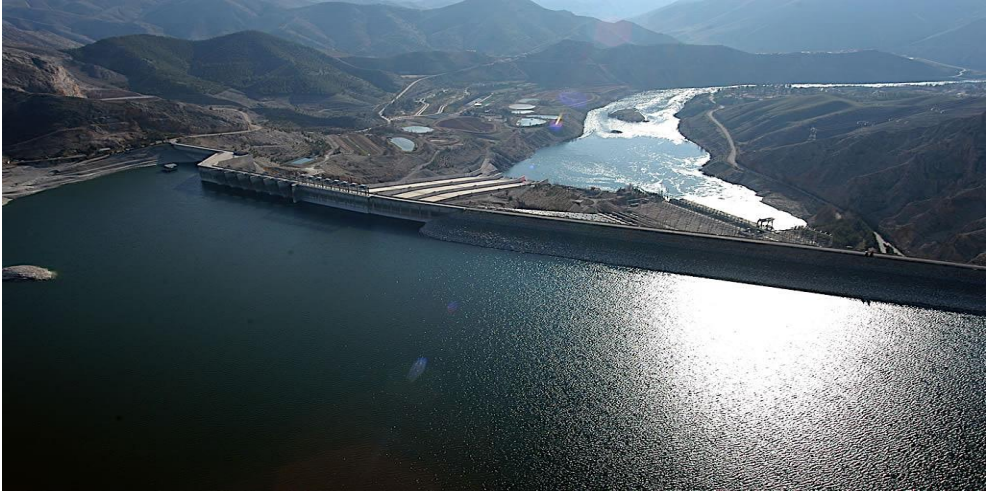
Fig. 1. General view of Keban dam (DSI , http://www.dsi.gov.tr/projeler/keban-baraj%C4%B1 )
