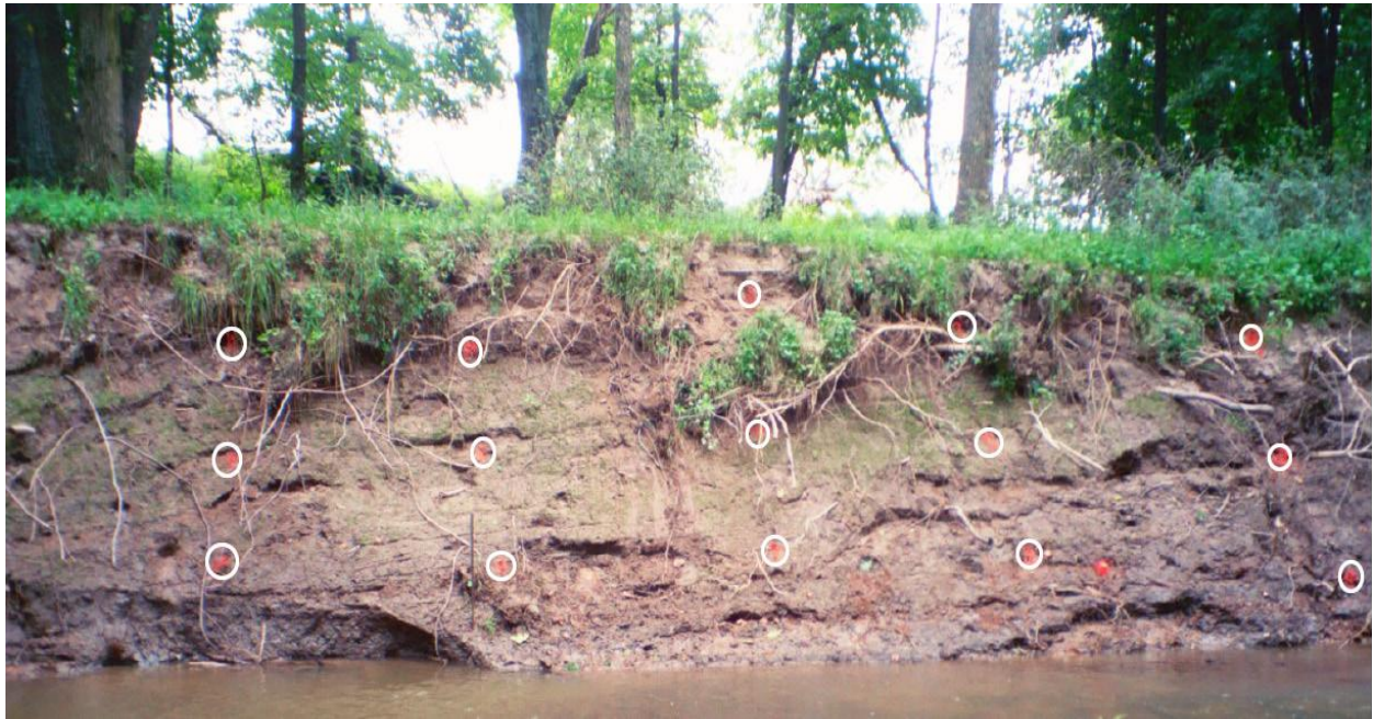
Figure 2. Pin arrangement on 3rd order stream. Banks are approximately 2.5m high.
