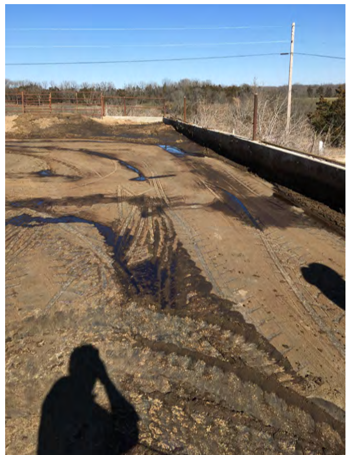
Figure 7a. Upslope view of sand lane.
