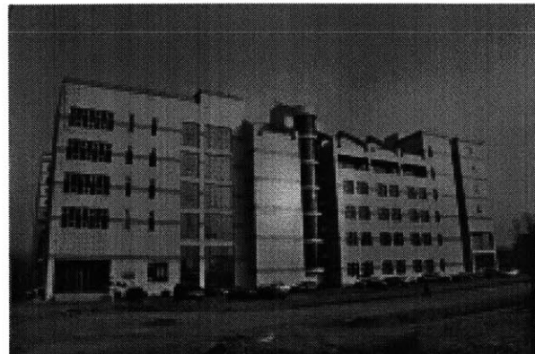
Office Building need to be demolished
