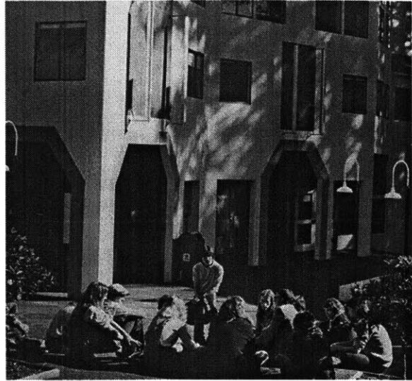
26. Designed by Charles W. Moore and finished in 1974.
