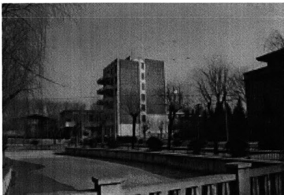
Academic Building need to be demolished
