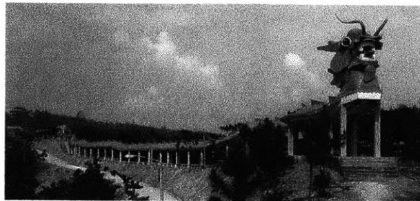
Fig. 30. A project in Kaiping City.
