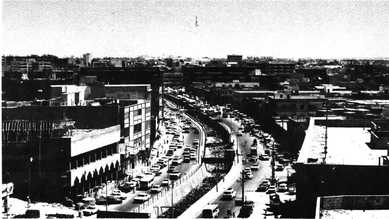
RIYADH, Saudi Arabia: (top) Batha Street, the main transportation and commercial spine with predominant walk-up apartment buildings.
