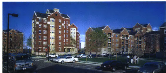
Figure 4-11: View II of Harbor Point (Source: MIT RVC Library)
