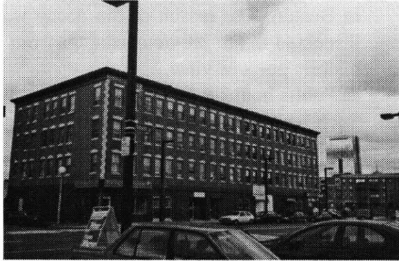
Existing building on the site (facade)
