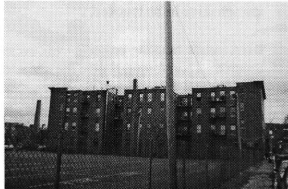
Existing building on the site (back)
