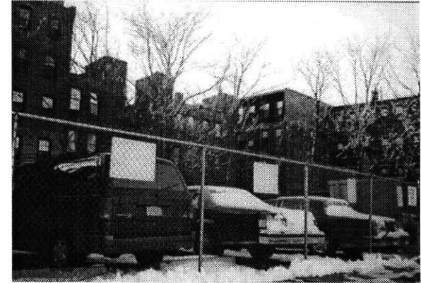
Site view showing the existing building and courtyard
