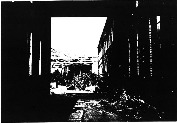
Figure 4-13. Photo of buildings and catwalks, July 1995. (photo by author.)
