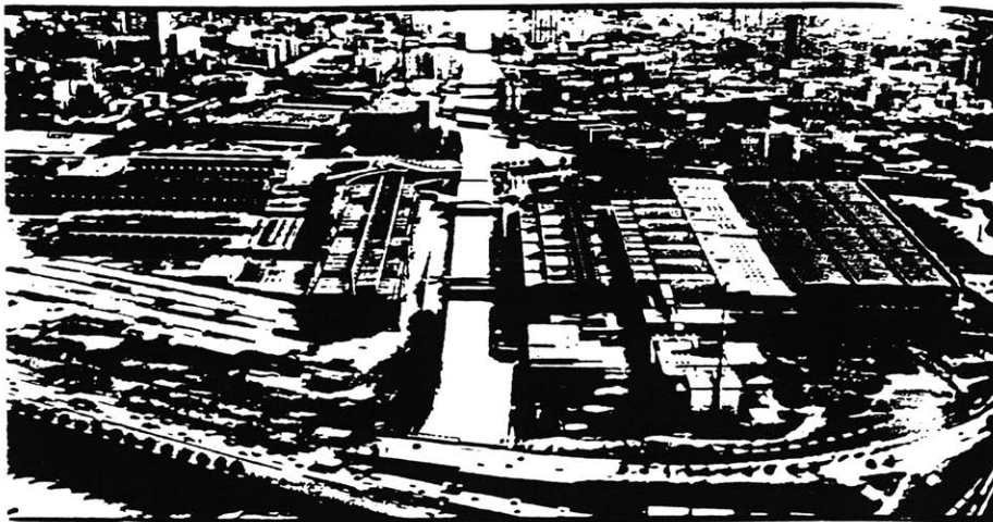
Figure 4-2. The former abattoir at La Villette with the canal running through the center of the site. (Boles, 1985.)
