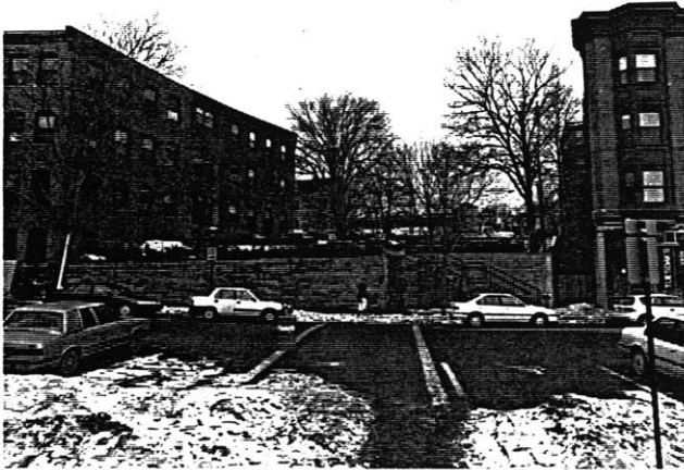
Fig. 23 Site from Station Street
