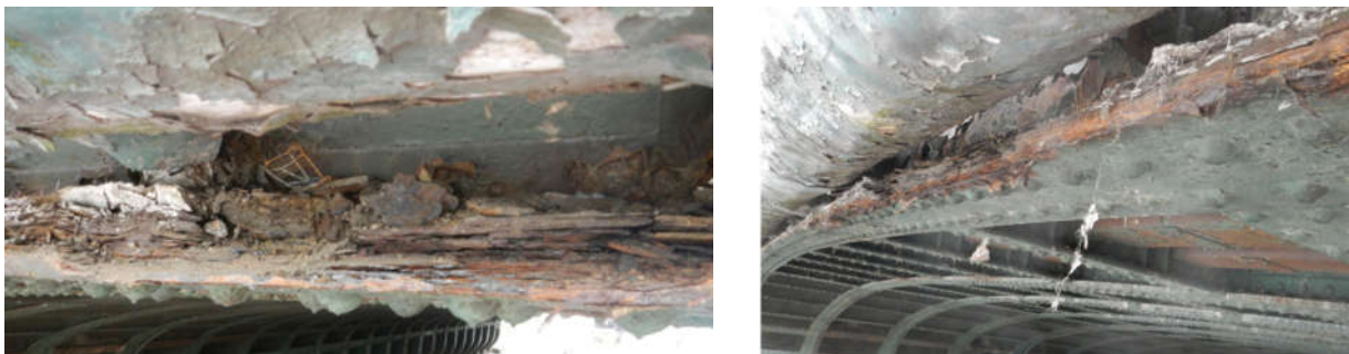
Fig. 8. Corroded rivets
