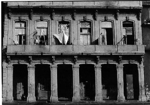
Facade of a typical 'apartamento' in the Malecon with barbacoas.
