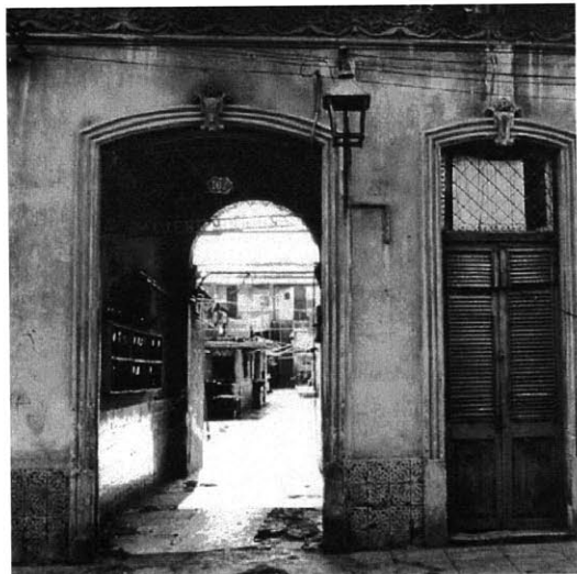
Street entrance to Modern Hygiene solar, Omoa Este, Cerro.
