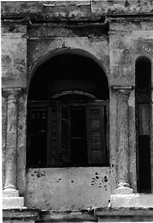
Typical view of a subdivided story. A barbacoa has been inserted. Bedroom space top level.
