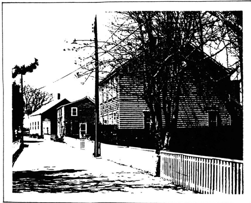
Fig. 2.2 Old Homes and Street
