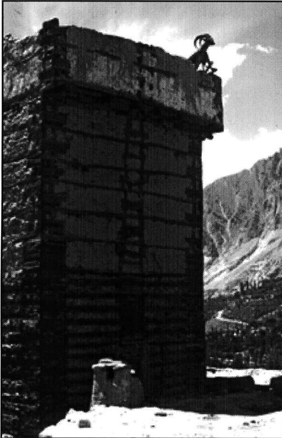
Figure 1.j Shingri Tower with Wood Cribbing Construction
