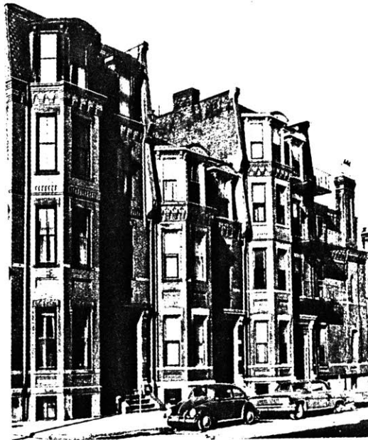
b. Facade of 7, 9, 11 Hereford Street and 435 Beacon Street, 1879, by R. S. Bither. Building permits for these houses indicate that they were planned as two stories with a mansard roof. Fourth stories were added for purchasers to two of the houses by the speculative builder before the row was finished.
