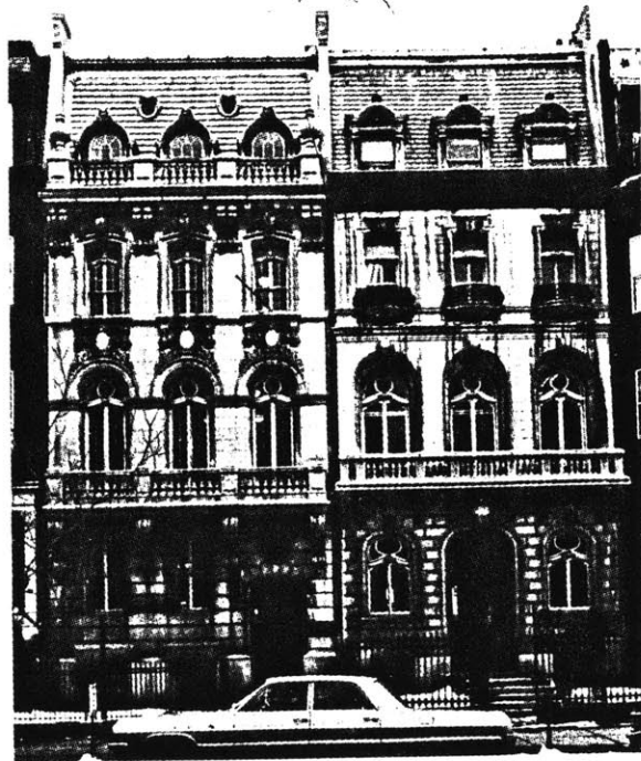
204 Facade of 128-130 Commonwealth Avenue. Constructed in 1882, the facades of these two dwellings were rebuilt about 1905 in the currently fashionable Beaux Arts Baroque manner.
