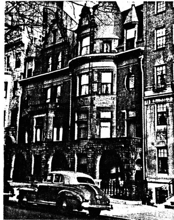
e. Facade of 176-178 Commonwealth Avenue, 1883, by Charles Atwood. The continuous line of bay windows and entrance porches would seem to violate property restrictions that limit projections beyond the building line to seven tenths of the lot width, but Massachusetts courts deemed these examples conforming.
