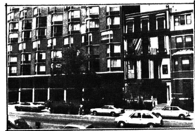
4.17 Detail of 4.16. Recessed primary plane at ground level results in discontinuity with adjacent houses.
