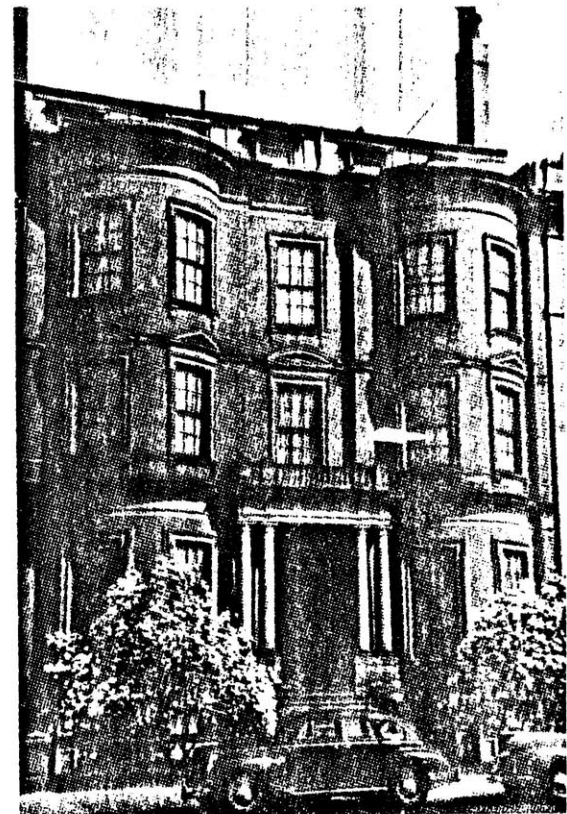
3.13b When the lot was wide enough to permit a central hall plan, the facade design was symetrical about the center.
