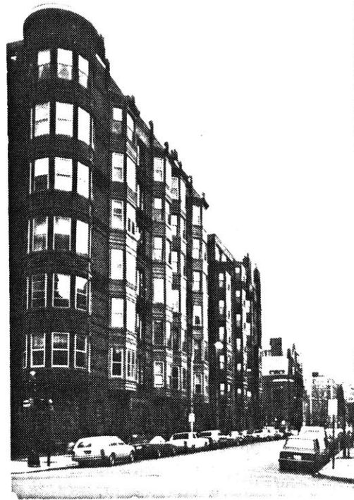
4.14 295 Beacon Street. Massive wall on a secondary street.
