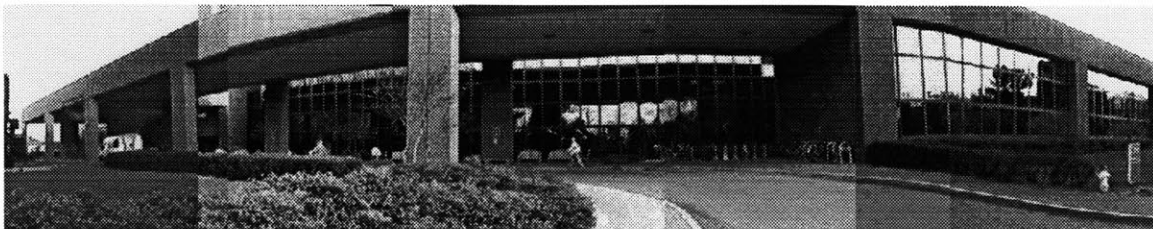
Figure 5.6: Clinical Center Complex entrance, apx. 180° Image. Note, image was produced by overlaying several digital video frames.
