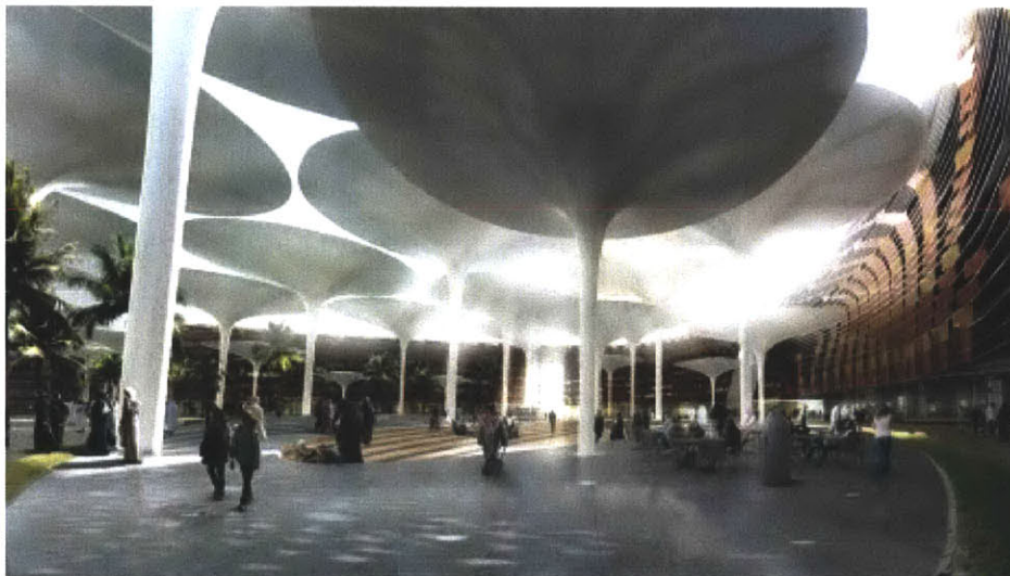
Figure 5.6 The PV canopy in Masdar
