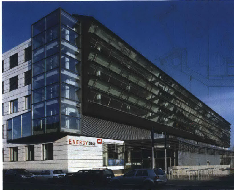
Figure 5.4 The PV shading façade in the ENERGYbase building Source: Waldhör, 2010/03
