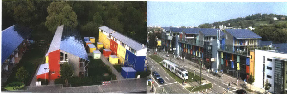
Figure 5.3 Photos of PV roofs in Vauban
