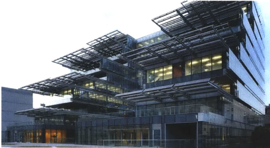
Figure 5.5 Extended PV eaves on Tsinghua University's environment and energy-efficiency building. Source: http://catalog.iguzzini.com/projectdetails.aspx?project=PRJIG_338
