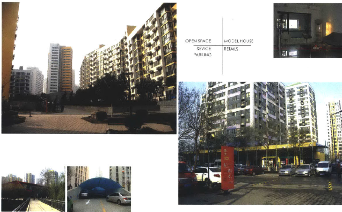
Figure 4.9 Photos of high-rise neighborhoods Source: ‘Making the Clean Energy City in China’, MIT research project, 2010
