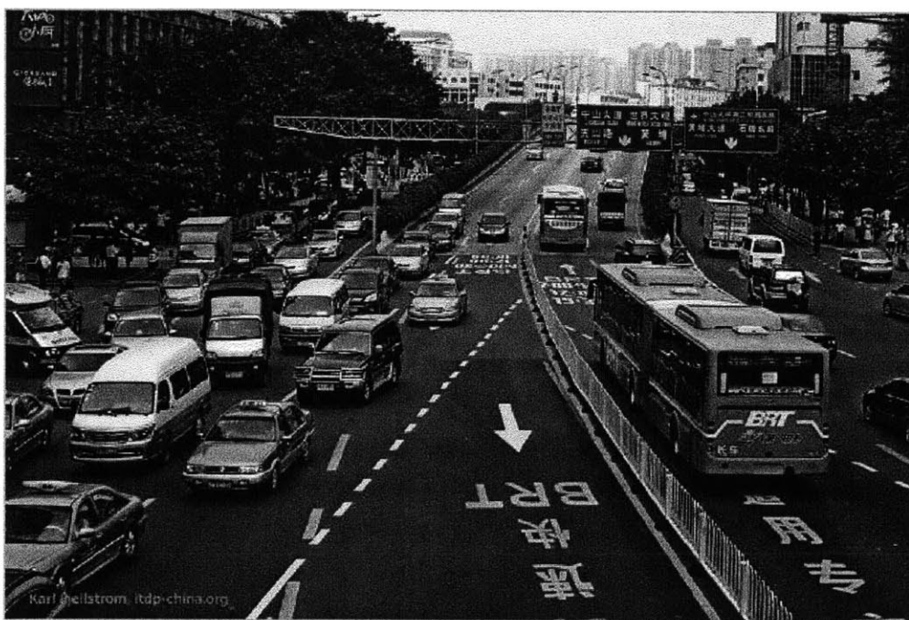
Figure 2.1-3: The entrance of a dedicated busway in Guangzhou
