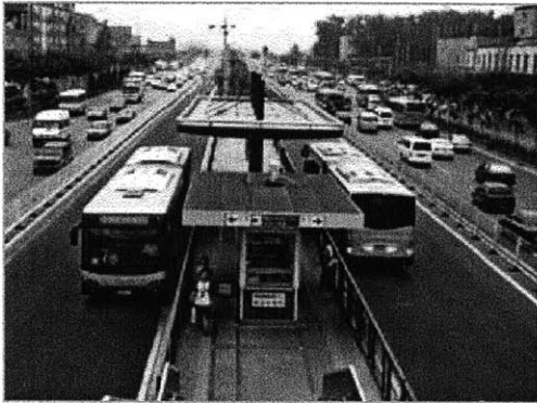
Figure 4.2-6: BRT stop in Beijing Source: [http://www.gztpri.com/xs-viewer.asp?id=13]
