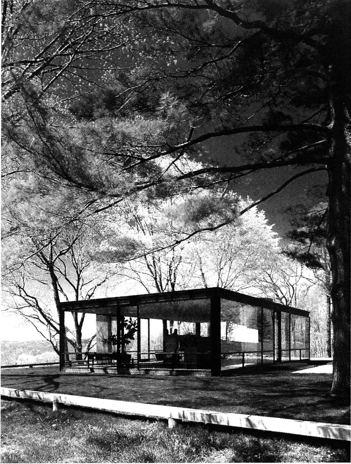
Fig. 13: Glass House, Philip Johnson, New Canaan, Connecticut
