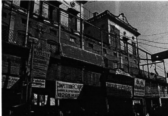
Figure 2.14: Image showing poor condition of buildings in Aminabad.
