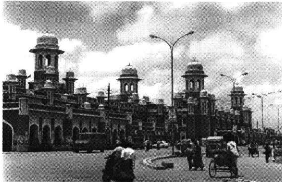
Figure 2.2: The Charbagh Railway Station, Lucknow.
