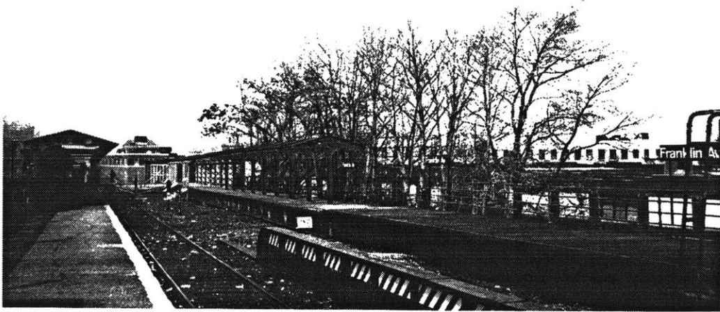
Photo #9: Franklin Avenue Station, Shuttle Terminus, April 1998 -- Undergoing Reconstruction
