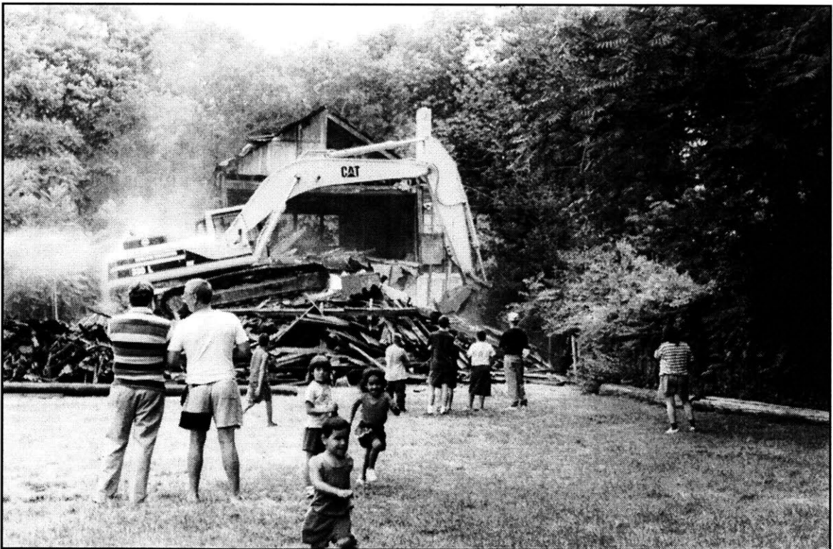
Site Photo-Stables Demolition August 1993 - Kim Kudrna
