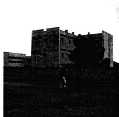
Figure 7: View of school
