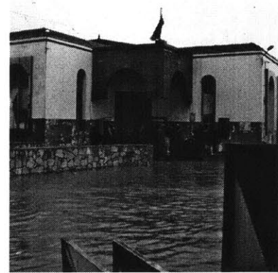
Figure 42: View of bus station in industrial zone (during flooding)
