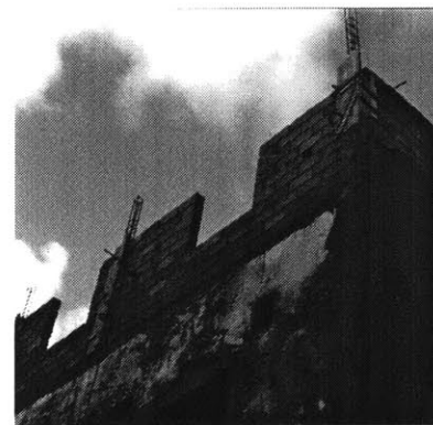
Figure 12: New floor addition to a house in the medina
