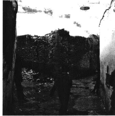
Figure 13: Collapsed house in the medina
