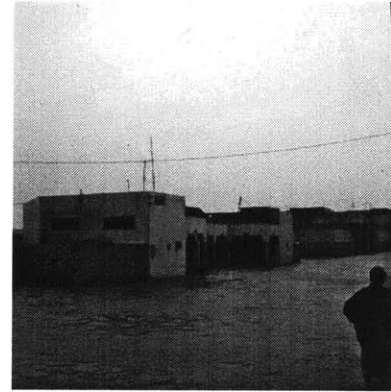
Figure 38: View of bus station in industrial zone (during flooding)
