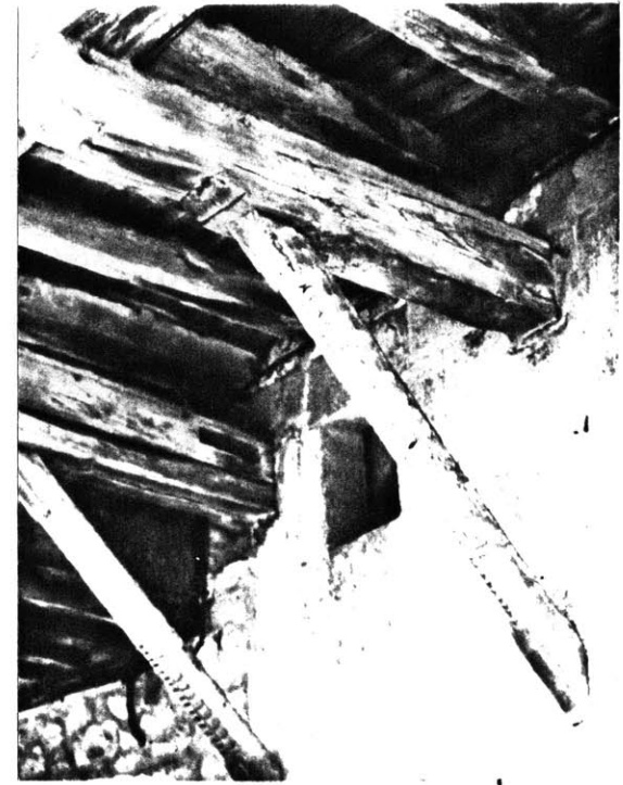
2: braced to wall
