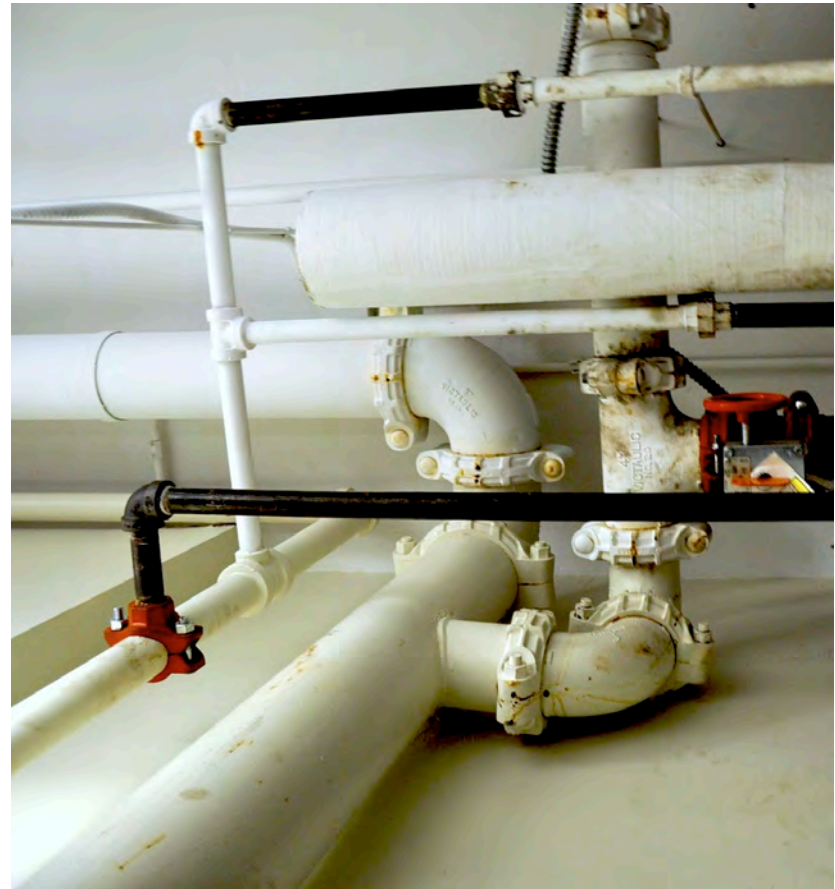
Building N51: interior view
