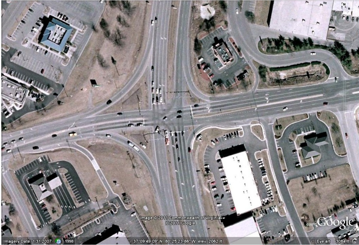
Figure 2-6: Satellite image of the Peppers Ferry intersection (US 460 and Peppers Ferry Rd, Christiansburg, Montgomery, Virginia 24073) taken from Google Earth. CICAS-V data from vehicles at Peppers Ferry intersection were used to test the algorithms presented in this chapter.
